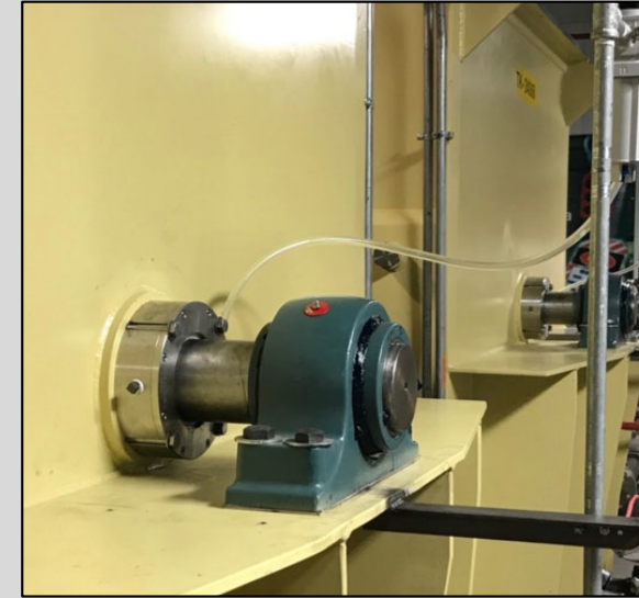
After: Inpro/Seal Air Mizer shaft seal installation
